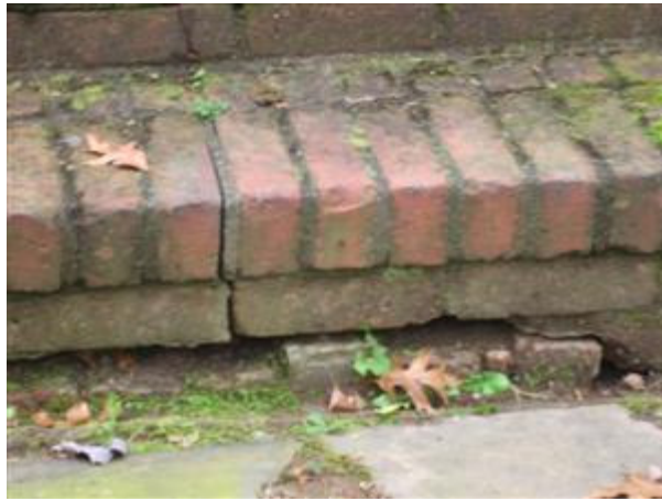
2.4 Picture 2 Right stair
