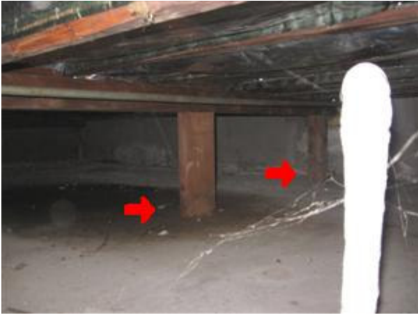
5.2 Picture 1 Temporary columns
