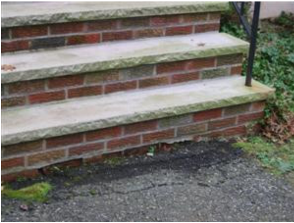
2.4 Picture 1 Left lower stair
