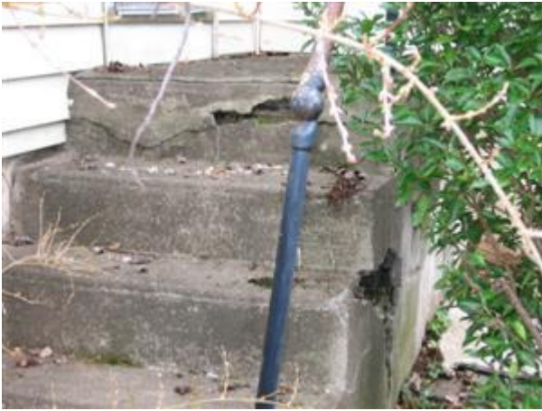
2.4 Picture 3 Side Entrance
